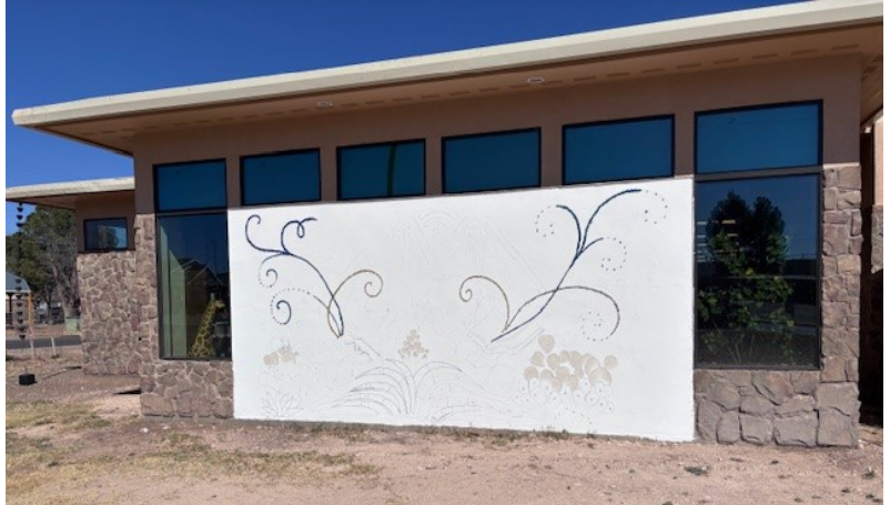
Mural in progress on south wall
