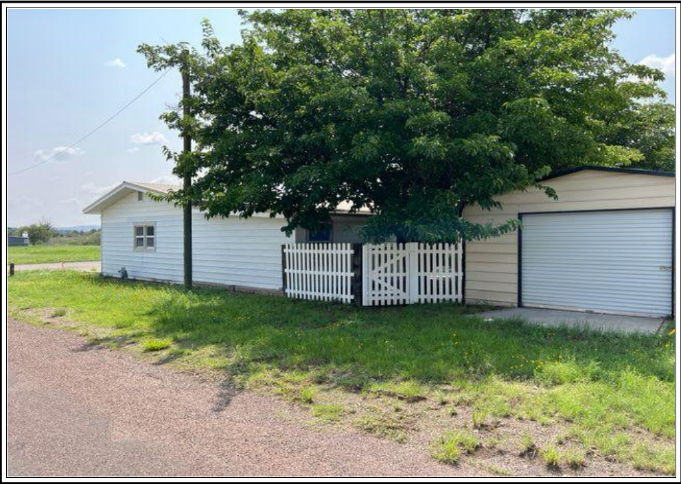
REAR OF SUBJECT PROPERTY
