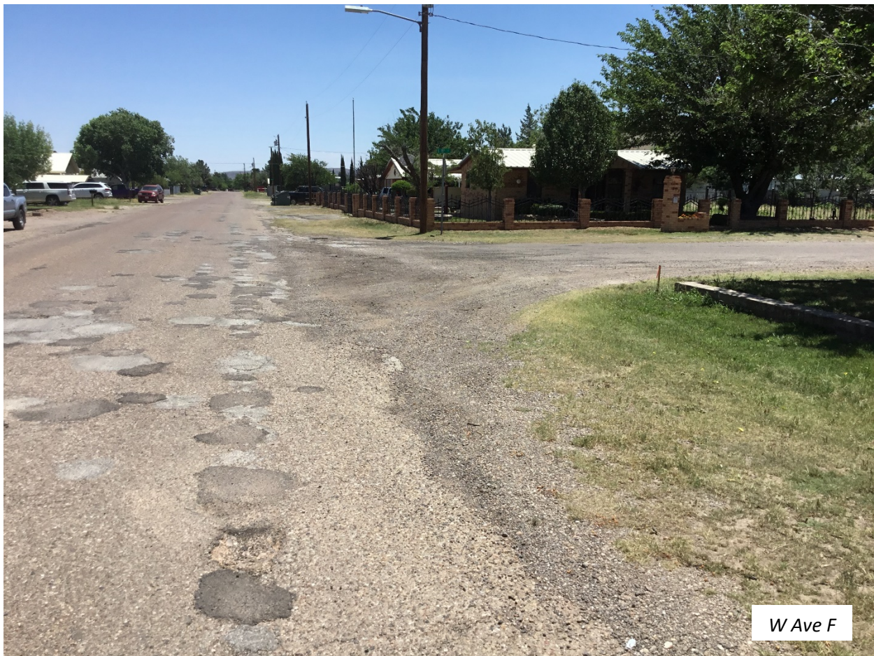
FIGURE 1-6 TYPICAL EXISTING CONDITIONS
