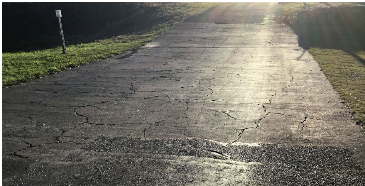
FIGURE 1-3 WEST MURPHY LOW WATER CROSSING PHOTO
